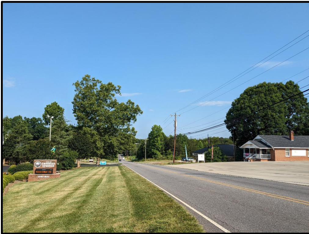
Photo 4: Highway 70 (Town Hall Location)
