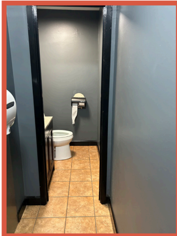
Doorways too narrow
