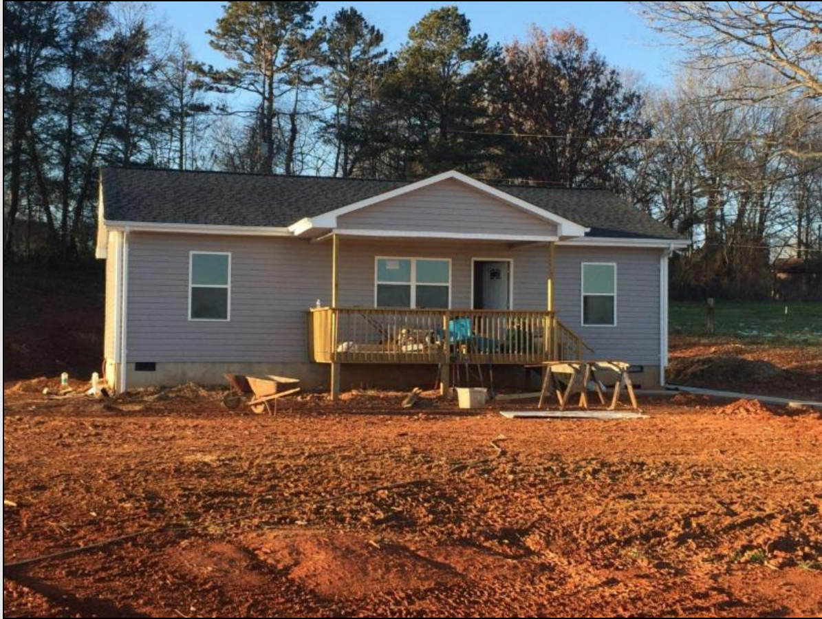
Construction of Alexander Habitat for Humanity Home, Cooksey Court Taylorsville.
